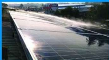
Solar Service and Cleaning
